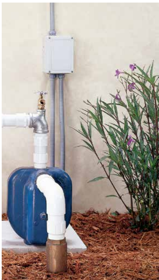
pump start relays
